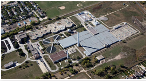
Photo: Winnipeg North End Sewage Treatment Plant (City of Winnipeg).
