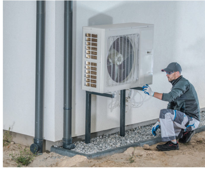
Photo: Heating and cooling technician installing heat pump (Dreamstime/Welcomia).
