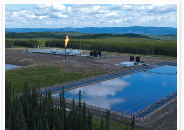
Photo: flare stack, North Montney Region (Peter McCartney).
