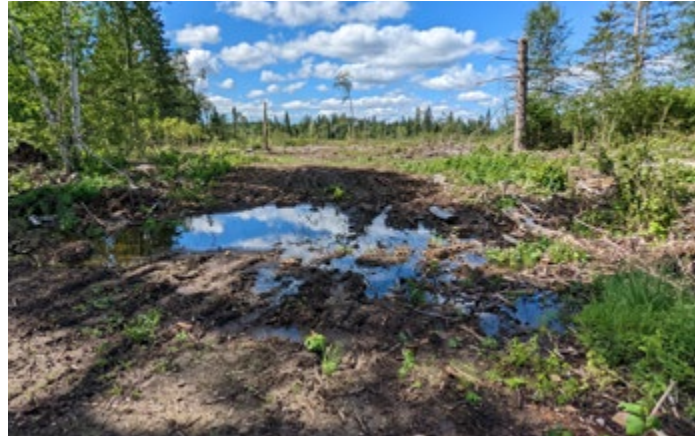
Water running over road at improper water crossing (cutblock JFL-806).
