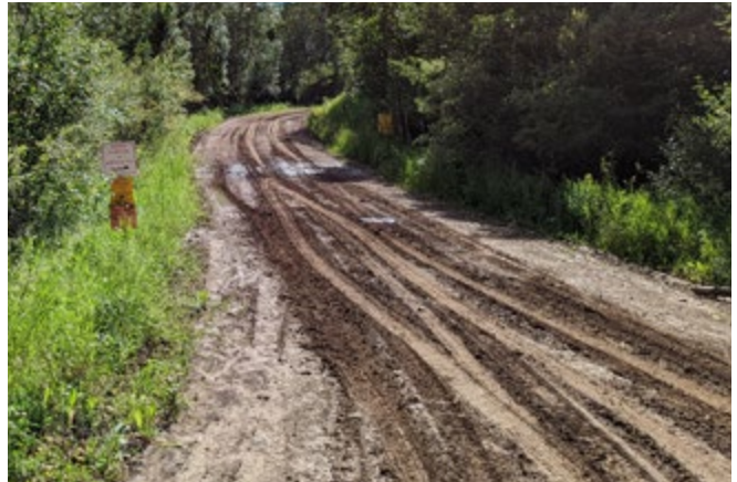
No gate on Island Lake logging road (road ISL-1A).
