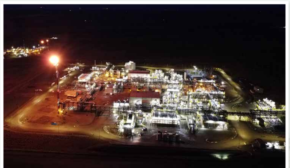
Photo: Ovintiv's Saturn Gas Plant in Farmington, B.C. (WC files).
