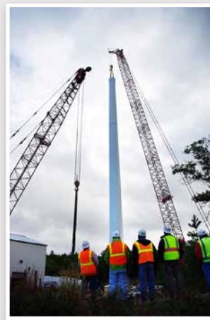
Photo: A wind turbine installation (WC files).
