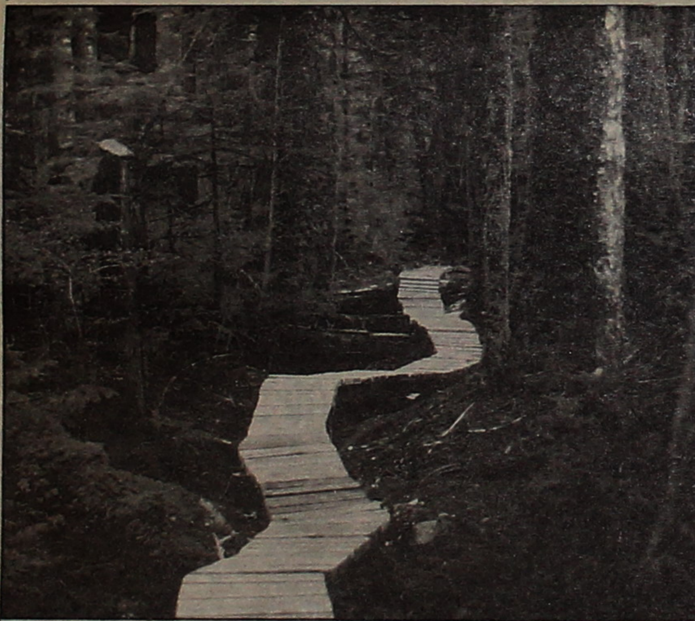
Boardwalk trail constructed by WCWC volunteers in the upper Carmanah Valley.
