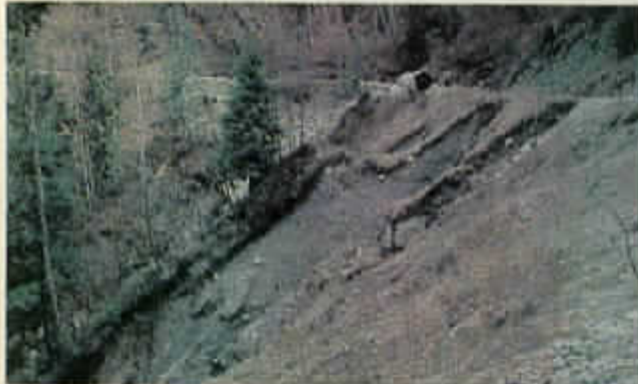
Capilano Watershed slide area along old logging road takes silt into the reservoirs.
