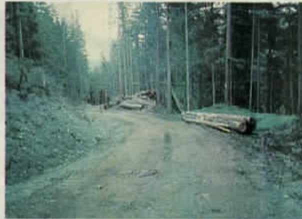
Meech Creek Road (rip/rap road through clay bed) built in 1992, Coquitlam Watershed.
