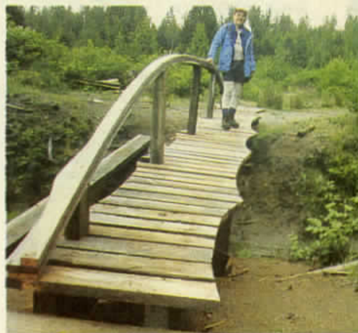
Completed bridge on trail by Ahousaht Village.
