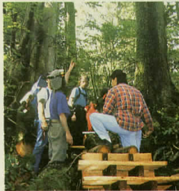
Boardwalking, Hole-in-the-Wall section of trail.
